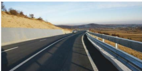
INITIATION OF THE INFRASTRUCTURE INTERCONNECTION PROJECTS
